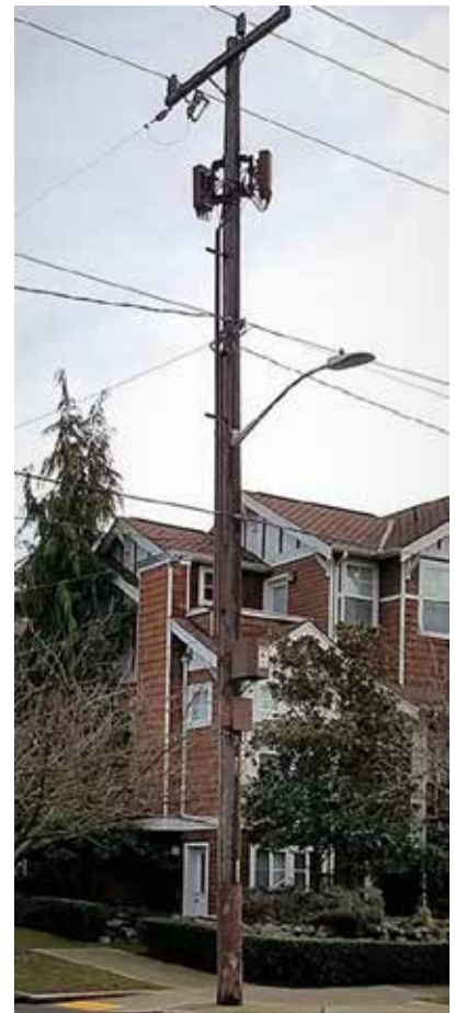
Image 1: Typical wood pole design with panel antennas
